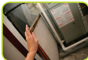
GAS HEATING SYSTEM
